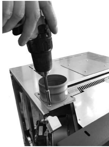
Fig. 47 - Secure the fitting
