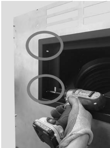
Fig. 66 - Trapdoor external fixing
