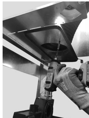
Fig. 65 - Flexible hose fixing
