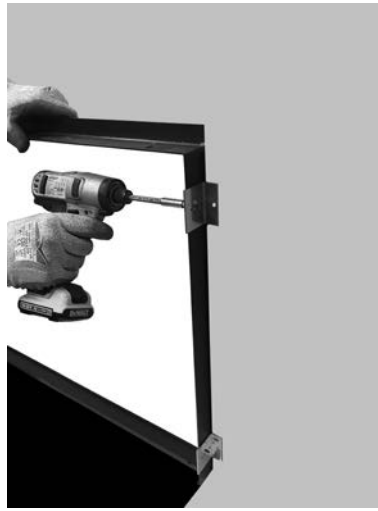
Fig. 73 - Rear fixing 1
