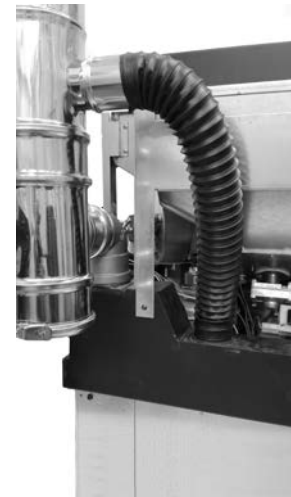
Fig. 77 - Combustion air connection
