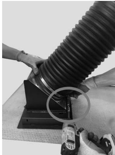
Fig. 62 - Tighten the clamp
