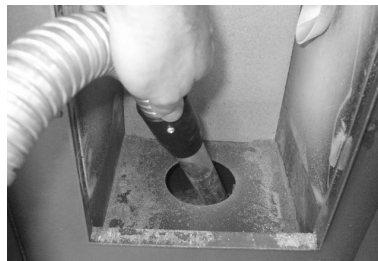
Fig. 39 - Burning pot box cleaning
